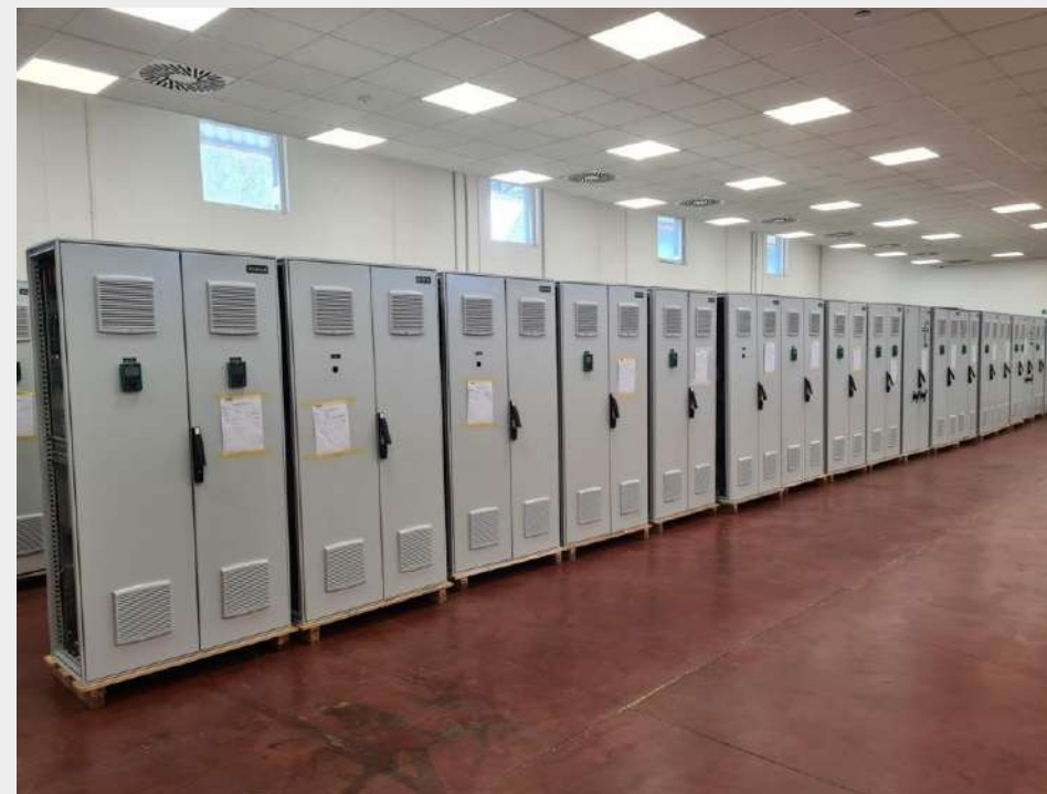
Motor Control Centre & PLC Cubicles
