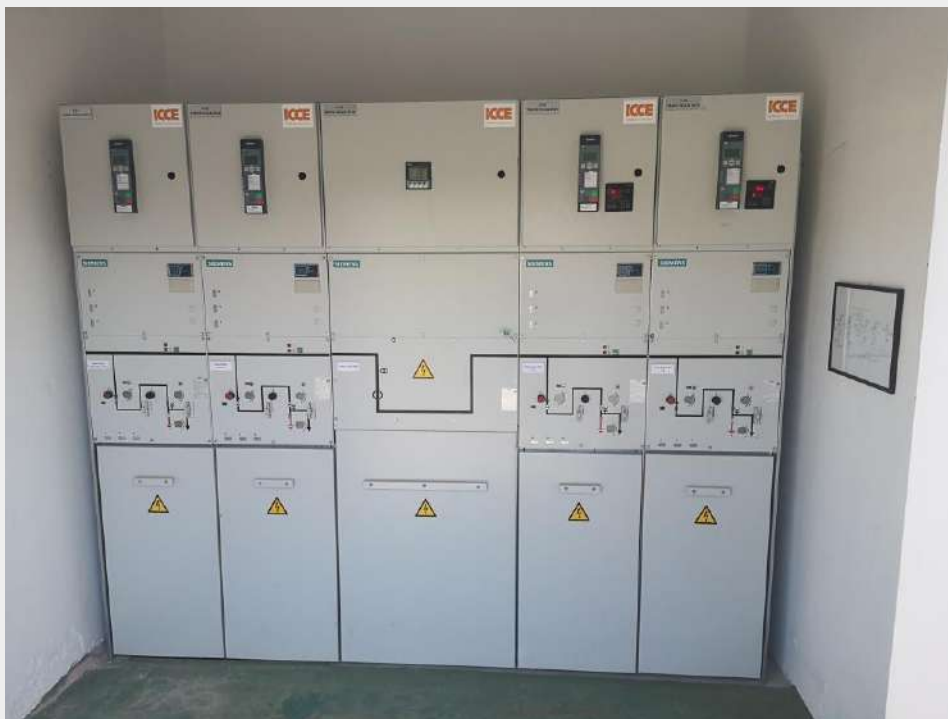
Medium Voltage Switchgear
