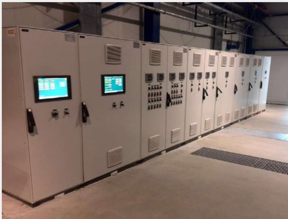
Motor Control Centre & PLC Cubicles
